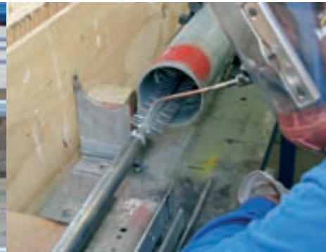
electrode joining
