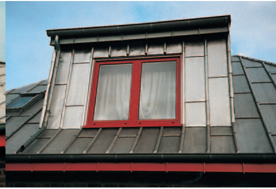
Complete roof covering with bleiPLUS
