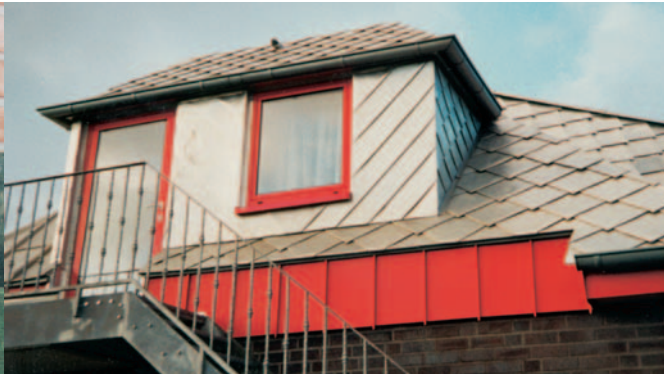
Façade cladding using shingle techniques
